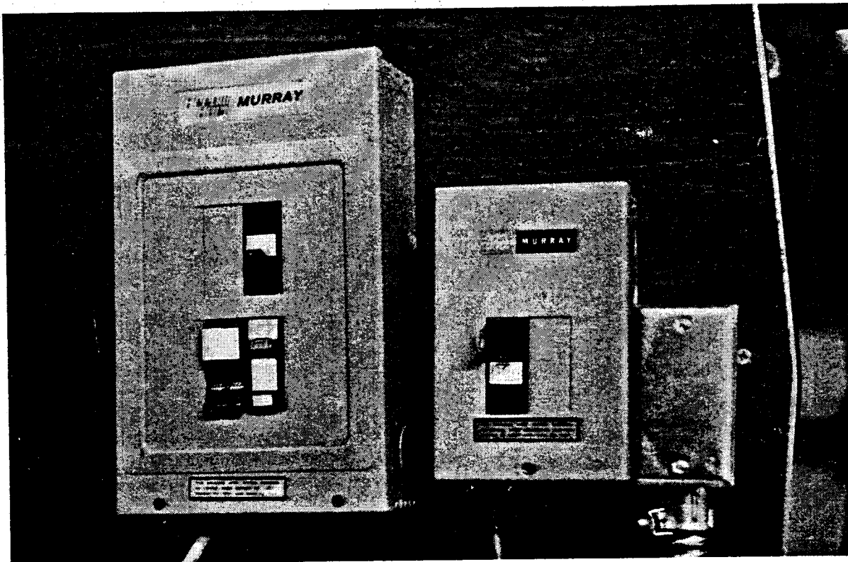
Figure 5-4. Typical Circuit Breaker Panels for Rear Bath Coaches
