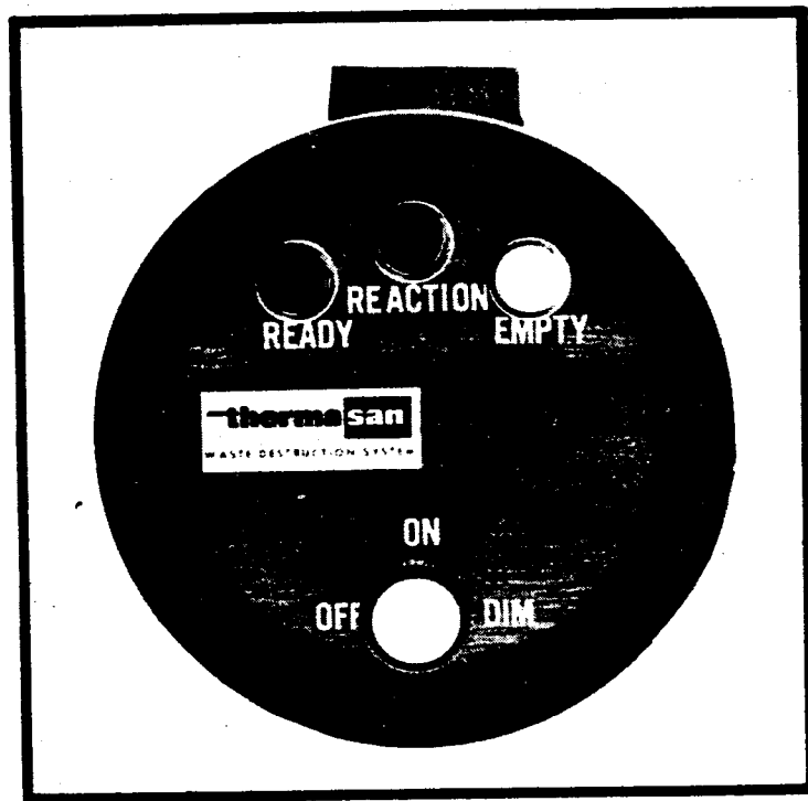
Figure 9-7. Thermasan Control Panel
